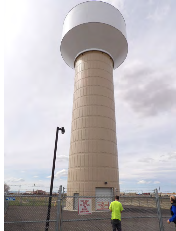
Great Falls - Gore Hill storage tank
