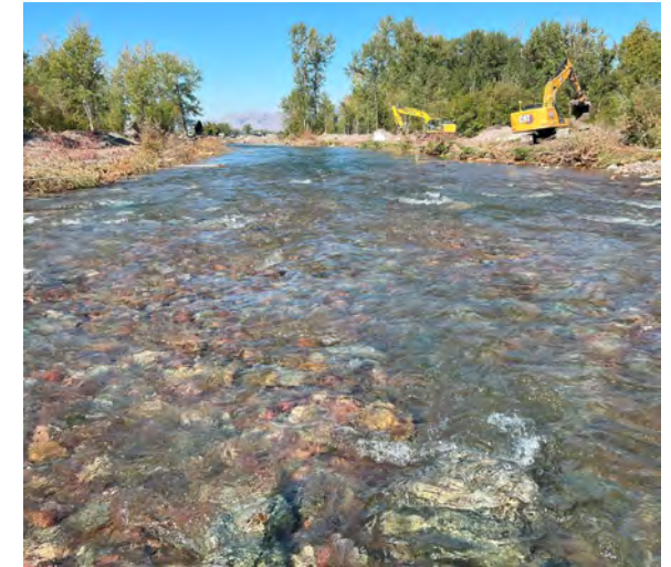
Flow in new channel (9/23/25)
