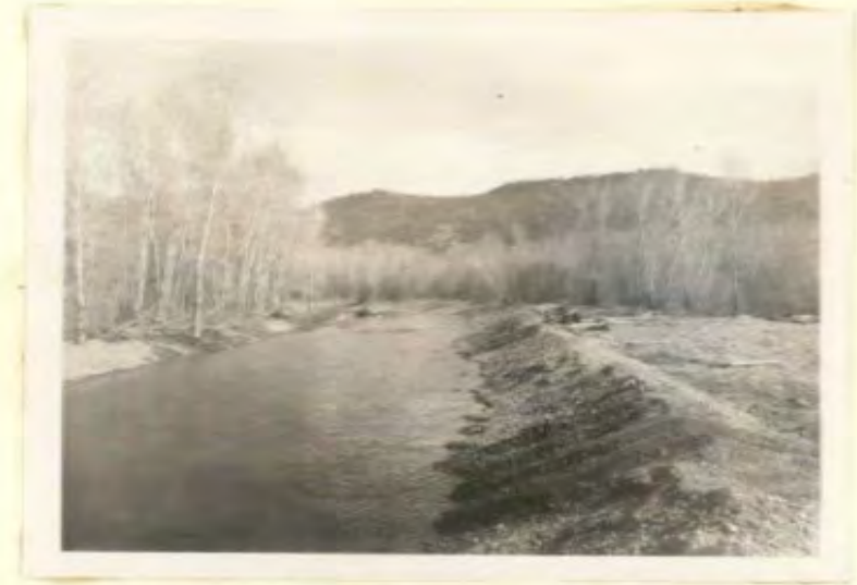
Material dozed from river bed forms a dike on both banks as protection from ice jams and to confine water during flood periods.
