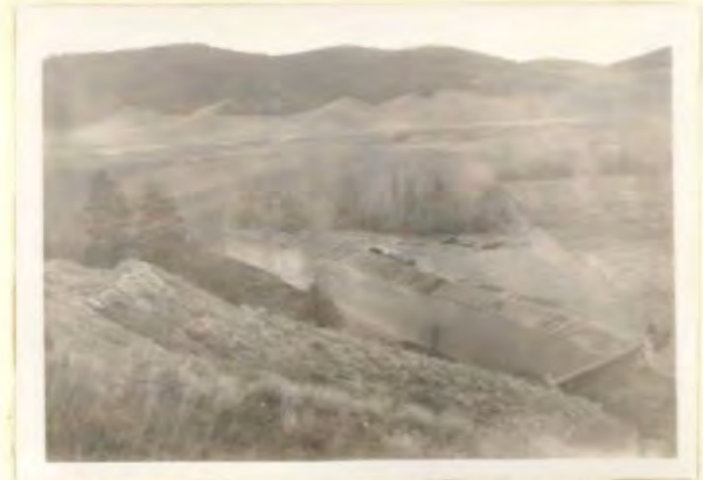
View from elevation showing No. 1 flood gate and boundary fence. Straight channel and diking is expected to protect flood gate and fence from ice jams and floods. This has been a bad spot.
